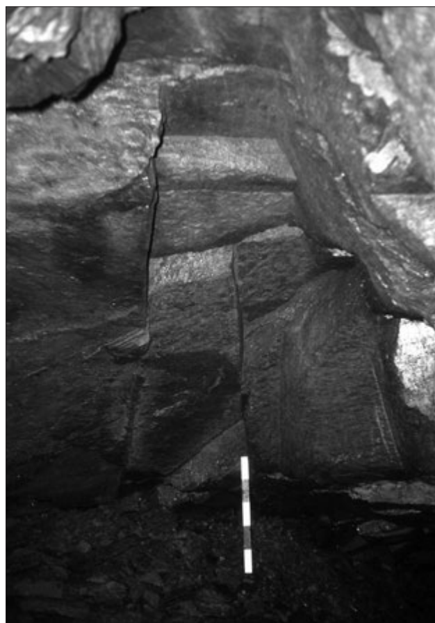
Fig. 15. Traces of early modern driving work at the end of the Venetian adit (Photo M. Strassburger).
